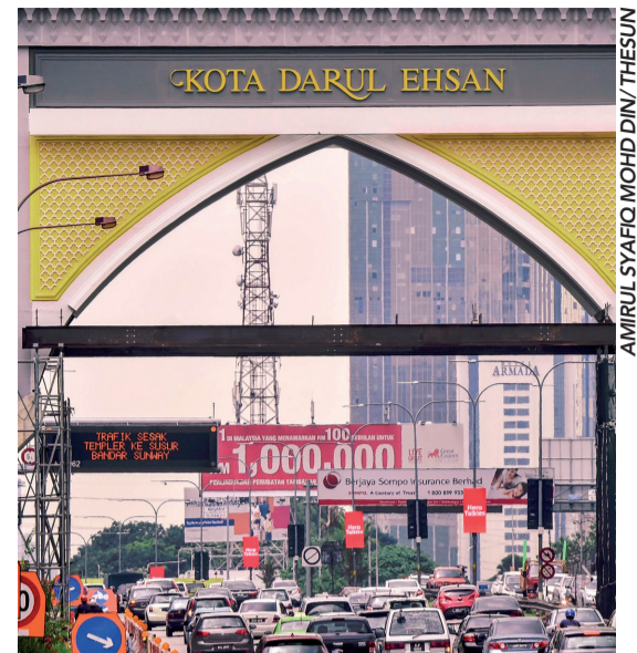
AFTER: The beam cleared of the construction materials.
